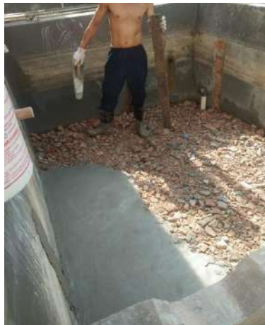
Proses pengecoran bak
